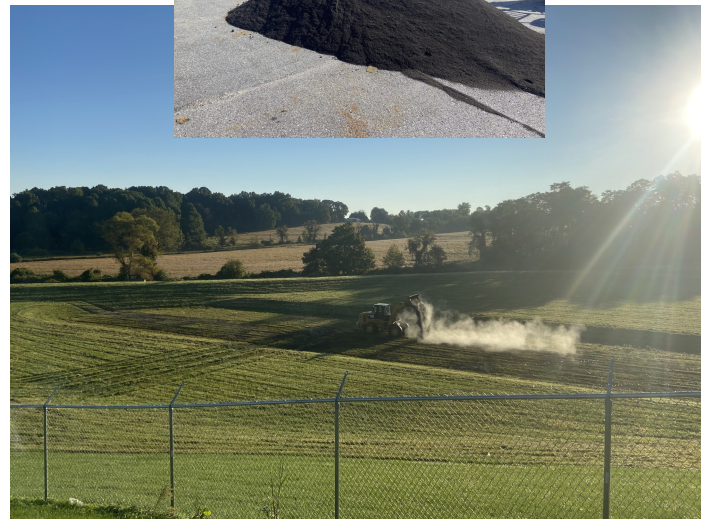
Iron rich media (above); media being added to the sand filter (right)
